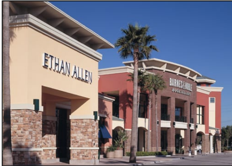
CPD: Commercial Planned Development Up to 6-story general commercial and large shopping centers
