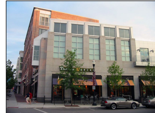
T4.8-4.9 (Urban General: Victoria Corridor) Up to 6-story workplace buildings and high-density mixed use
